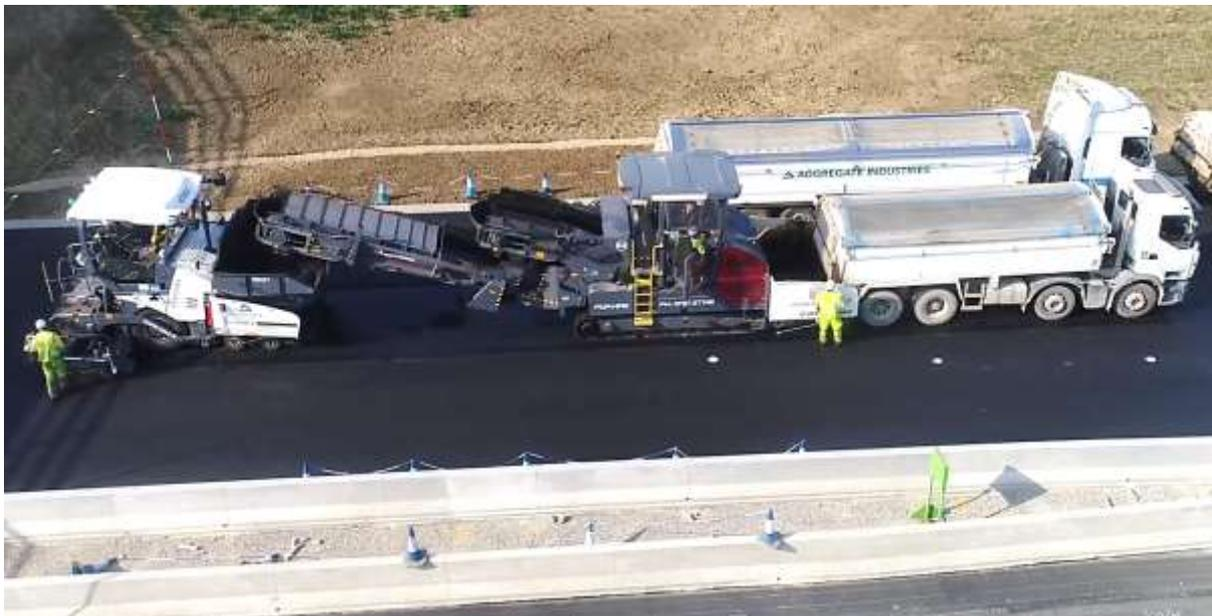
**Section 3:** The final layer of road surface is now being laid (see picture above) and white lines and other road marking will begin in the next few weeks. The last bridge over the A14 Huntingdon southern bypass, at New Barns Lane, is now structurally complete, with kerbing underway ahead of surfacing.
